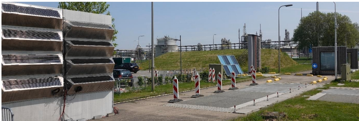
Fig. 2. Outdoor test facility for IIPV, BIPV and window innovations at the Brightlands Chemelot Campus in Geleen.
